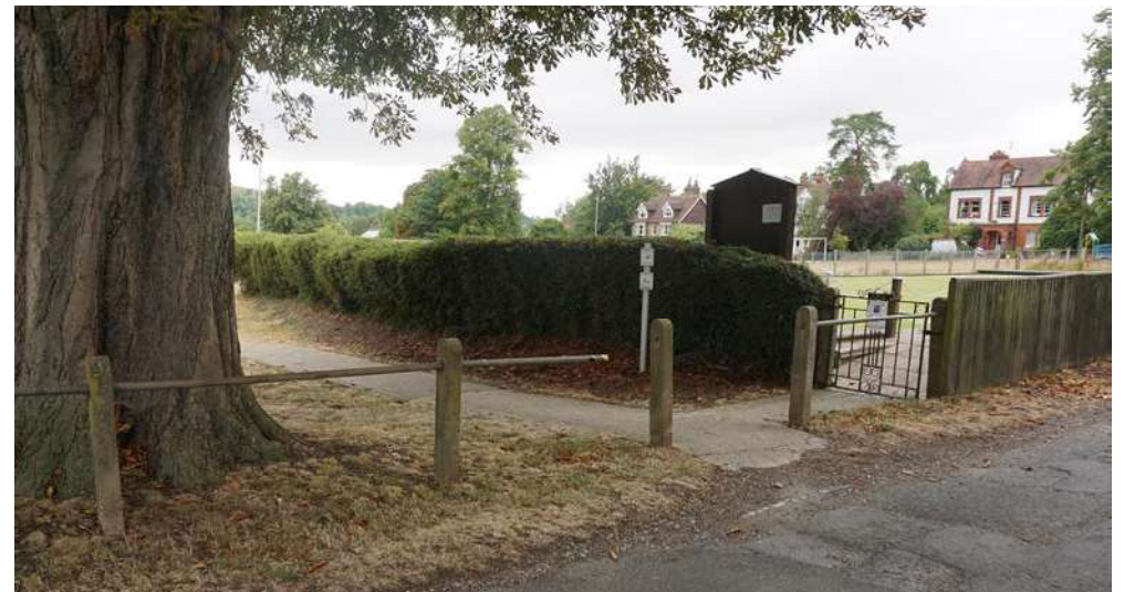
G2.7 - damaged perimeter fence gives a poor impression
