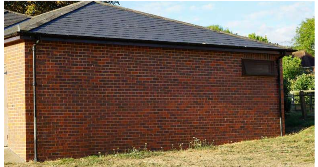
G1.4 Rear face of the pavilion is unwelcoming
