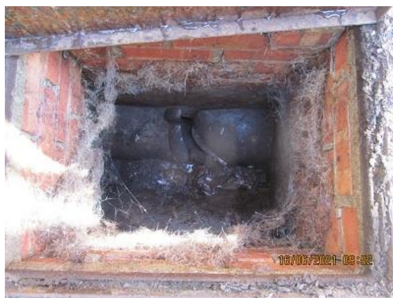
Photo 42 – Drainage inspection chamber
