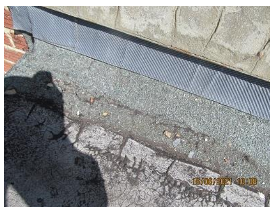
Photo 18 – Cracks to felt verge
