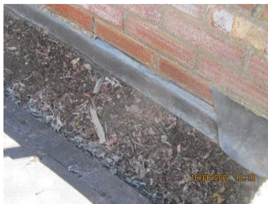
Photo 16 – Blocked parapet gutter/flashing pulling from masonry
