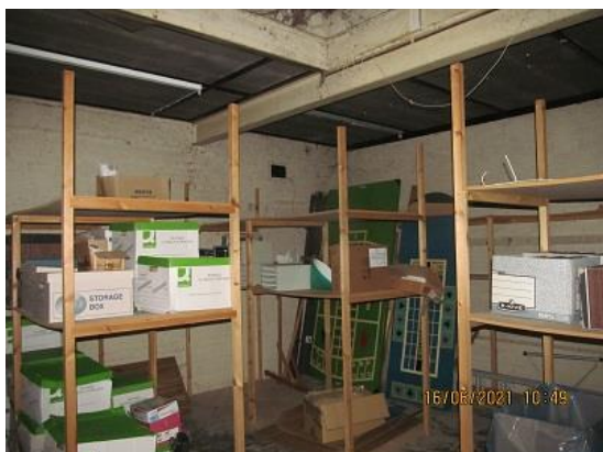
Photo 30/30A – Rear Store Room/fibre cement ceiling & water ingress high level
