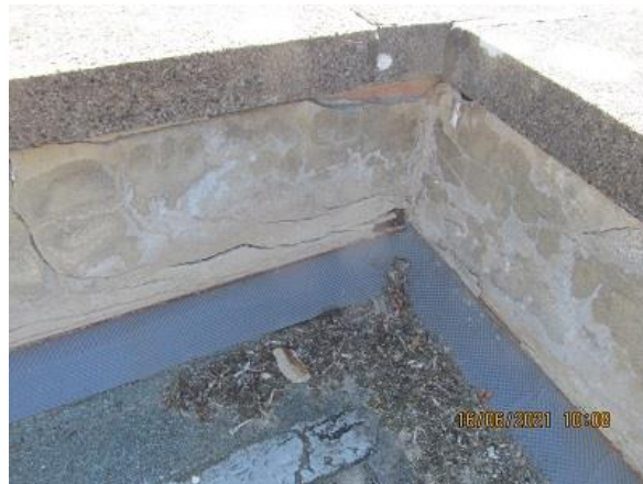
Photo 19 – Cracked and addled rendering inner face parapet
