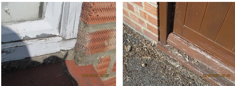
Photo 4/4A – Rot window sub frames; loose weatherboard
