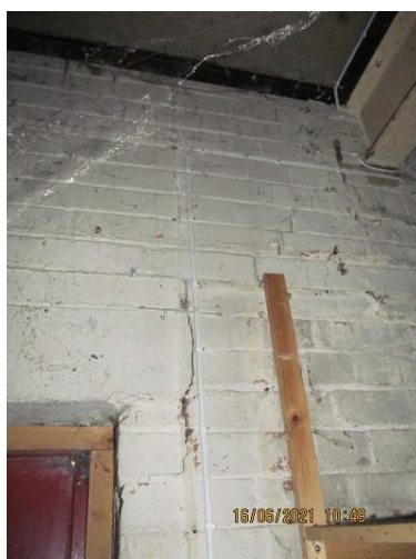
Photo 31 – Cracking above rear door head
