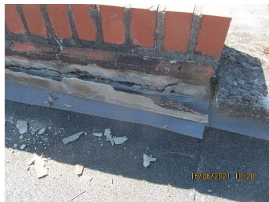
Photo 21/21A – Cracked, addled parapet rendering and corroded angle bead
