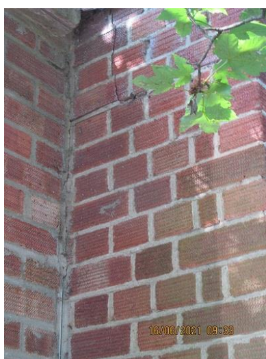
Photo 6 – Cracking between front infill extension and original
