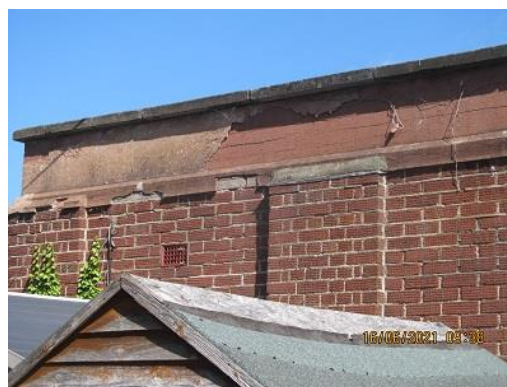
Photo 10/10A – Rear left elevation/addled and cracked rendering
