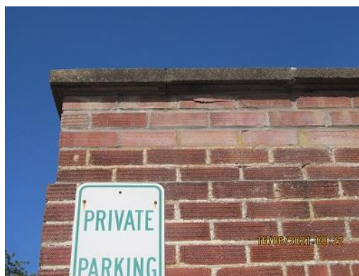
Photo 3 – Staining below front parapet; laminating bricks
