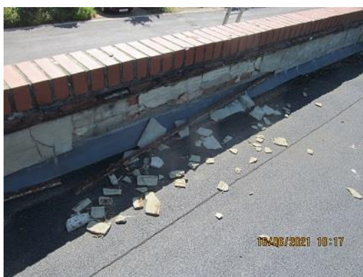
Photo 21/21A – Cracked, addled parapet rendering and corroded angle bead
