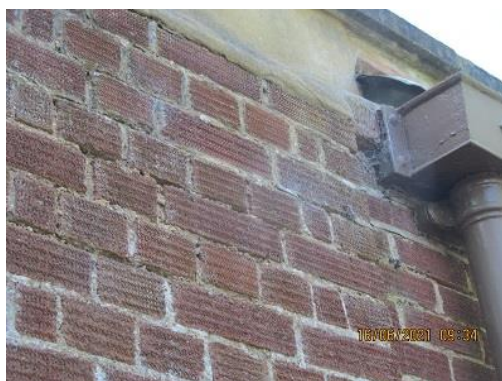
Photo 7 – Open jointed brickwork
