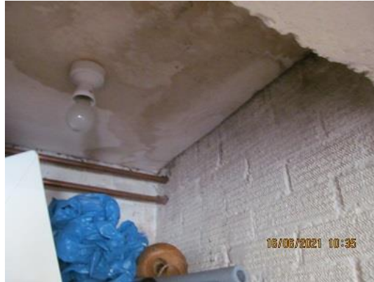
Photo 24/24A – Cupboard/damp and black spot mould ceiling
