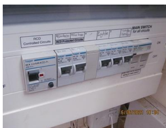
Photo 32/32A – Electric meter/distribution board
