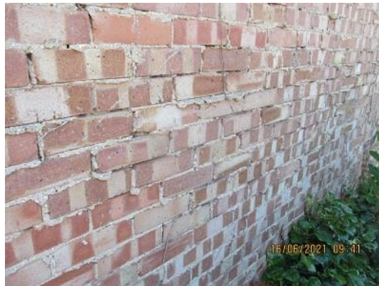
Photo 14 – Open jointed rear clay common brickwork
