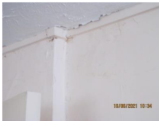
Photo 23 – Damp staining and water damage office ceiling
