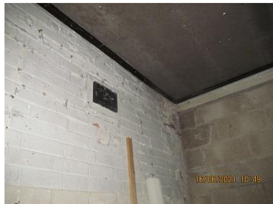
Photo 30/30A – Rear Store Room/fibre cement ceiling & water ingress high level
